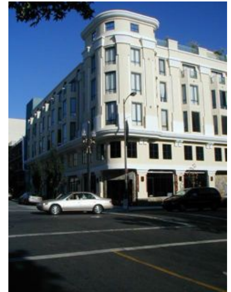
The ARTech Building Berkeley, CA 2002
